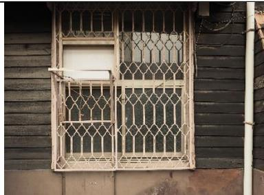
DW-004-鐵窗面漆剝落、鐵件鏽蝕
